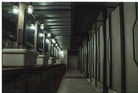
TOP LEFT: Drab bathrooms subdivided by cement boards and VMS frames
